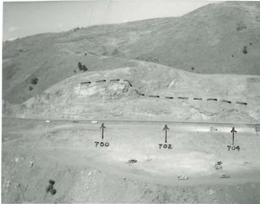
Figure 1. Boundary between rippable and non-rippable material in cut section between Stations 698 and 706. Compare with velocity boundary shown on Plate 5.
